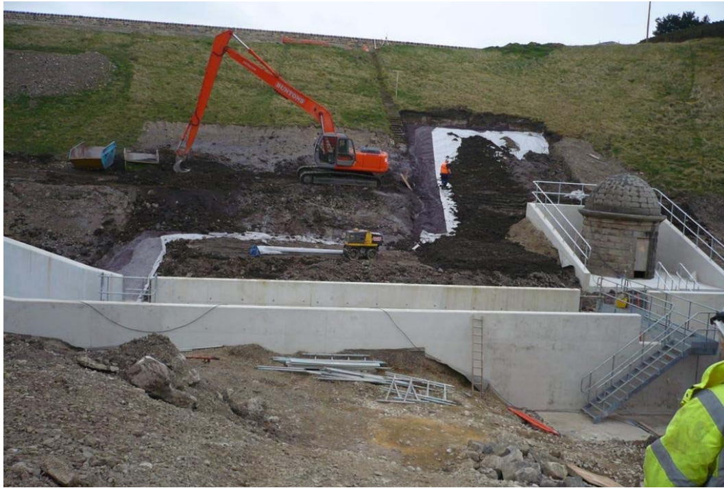
Figure 22 - Downstream filter berm installation
