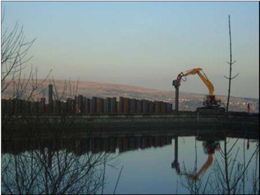
Figure 23 - Sheet pile installation
