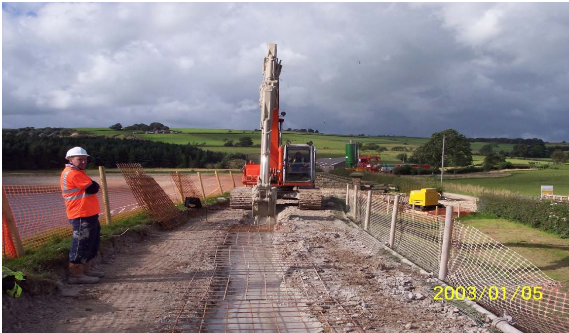
Figure 25 - Slurry trench installation
