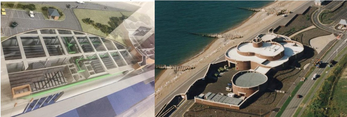
Figure 1: Eastbourne wastewater treatment works cross section showing primary and secondary treatment works below public car park
